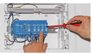
For the sustainable Wireless Building actuators should be installed as modular devices in distribution cabinets – regardless of the nature and use of the building.
